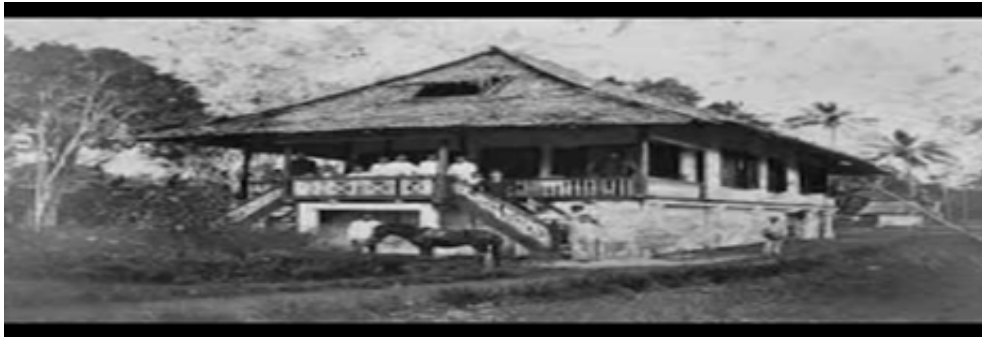
Figure 6. The Old Minahasa Stilt House
